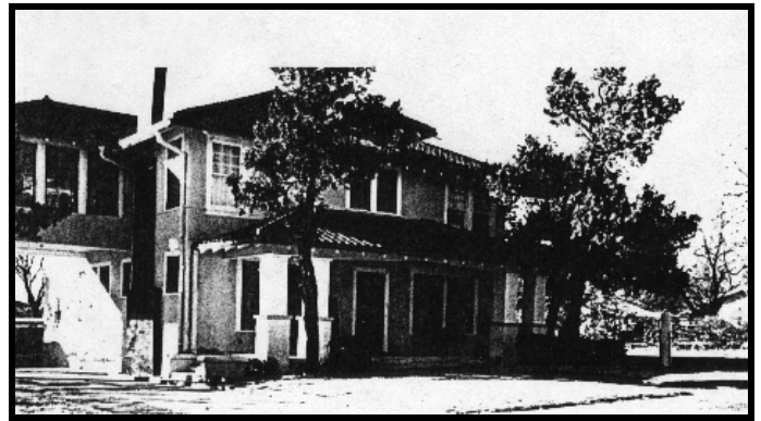
FRONT VIEW - PROBABLY AROUND 1997 FOLLOWING RENOVATION
